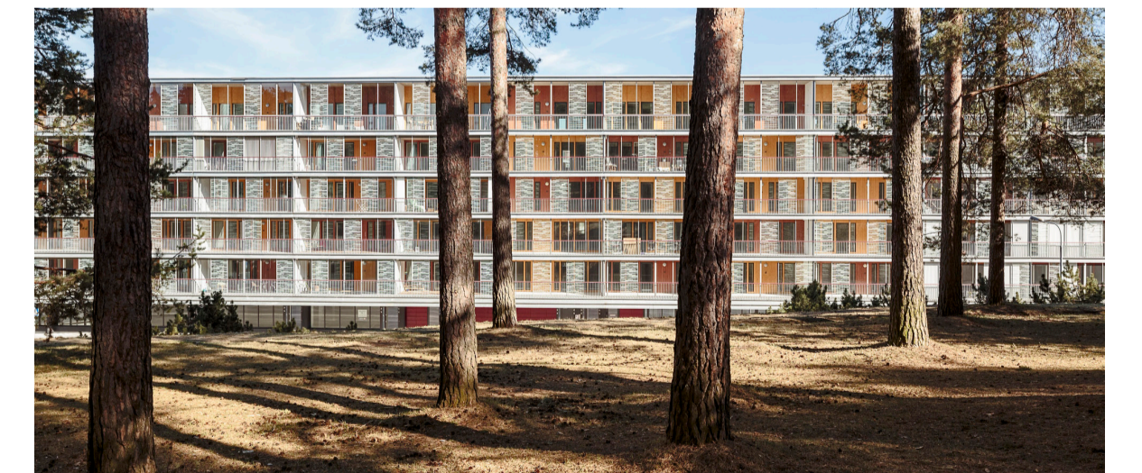
Harjunkulma Housing, Denmark Kirsti Siven+Asko Takala Arkkitehdit
